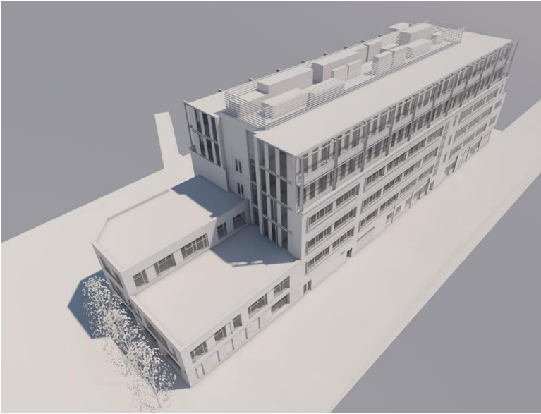
Image 18. Part 2, part 3 storey (BRE compliant) extension over car park.
