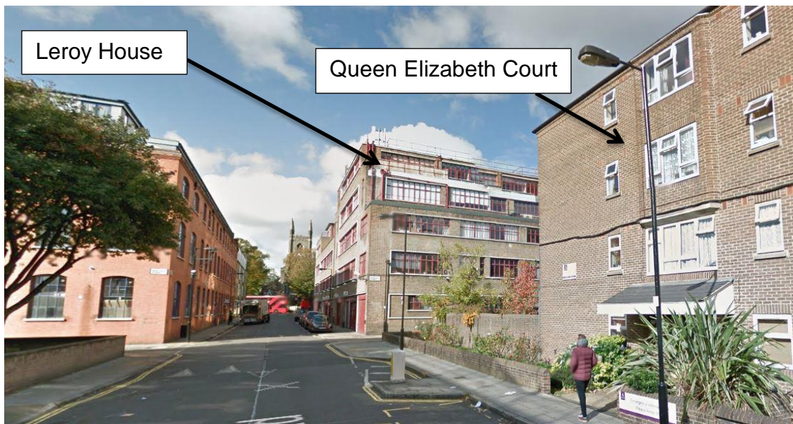
Image 15. Eastern elevation of Leroy House viewed from Dove Road
